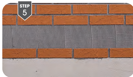
Arrange the first & fourth row of slips along the lines.
