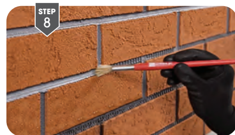
The adhesive must slightly cover the edges of the slips. Smooth the adhesive in the joints with a damp, (but not wet) brush.
