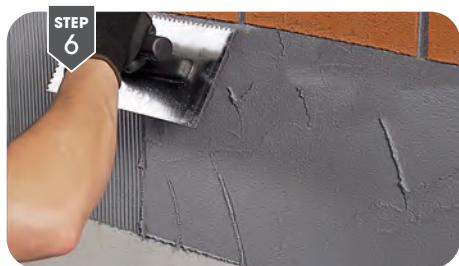
Apply adhesive between the lines with 4 x 4 notched trowel.
