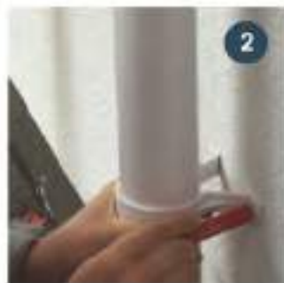
Mark the wall
